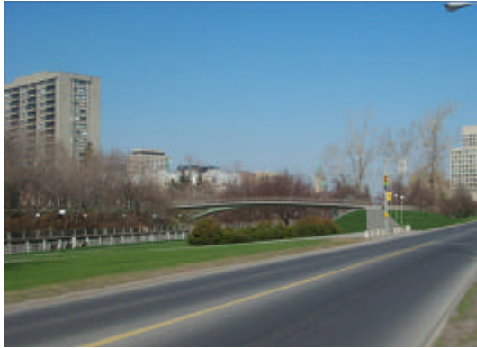
Figure 133: Rigid Frame Bridge (Single Leg)
