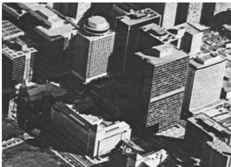
Figure 10: Aerial View of Place de Ville (Ottawa Views, 1993)
