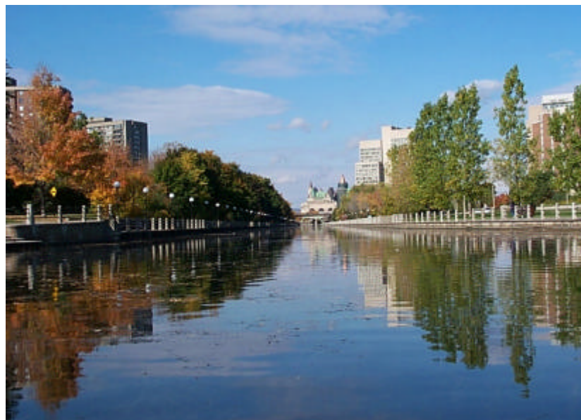
Figure 129: View of Rideau Canal, looking north
