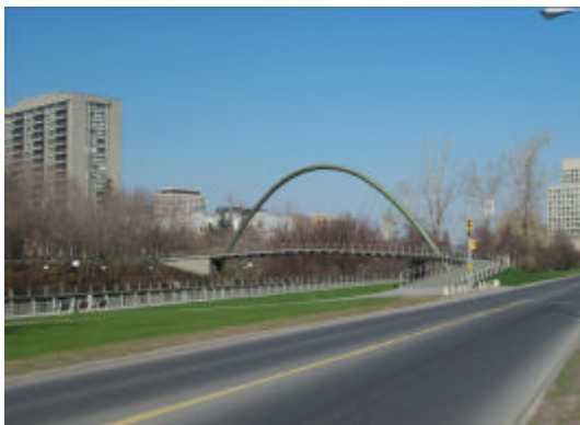
Figure 137: High-Level Curved Single Arch Bridge
